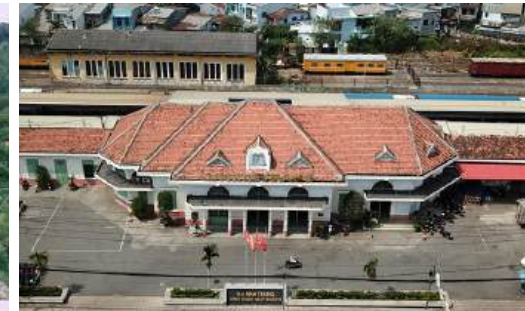
5 Nha Trang Rail Station
