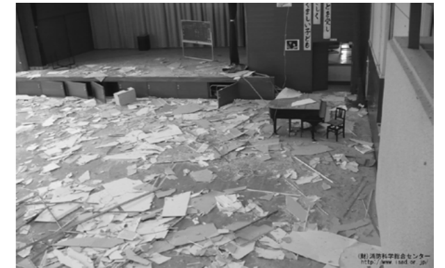
Figure 1. In this school gymnasium large amounts of ceiling materials fell off (the Great East Japan Earthquake, Sakae-mura, Nagano prefecture) 1)
