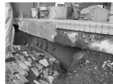
Figure 7. Piping passing through inlet portion of the building
