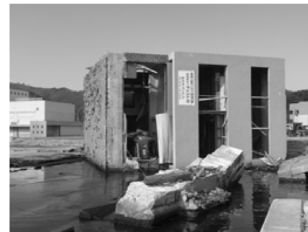
Figure 3. This overturned building in Onagawa-cho, Miyagi prefecture will be preserved as a demonstration and reminder of the threat of a tsunami. It will also help in the investigation of the tsunami and its effect on the building.
