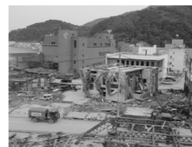
Figure 5. An old three story reinforced concrete building which was floated by the water, moved, and overturned, and a new reinforced concrete building with minor damage
