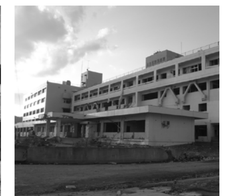
Figure 4. Shizugawa Public Hospital (Miyagi prefecture), which had finished a seismic retrofit, suffered from the tsunami which was much stronger than the Chilean Tsunami.
