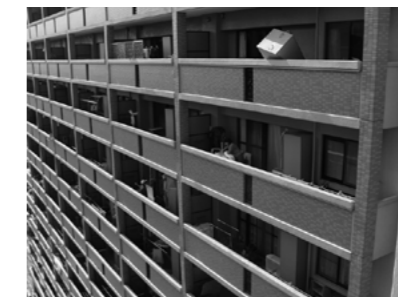
Figure 2. Storage type water heaters, etc. placed on balconies were damaged by shaking and left leaning or out of alignment.
