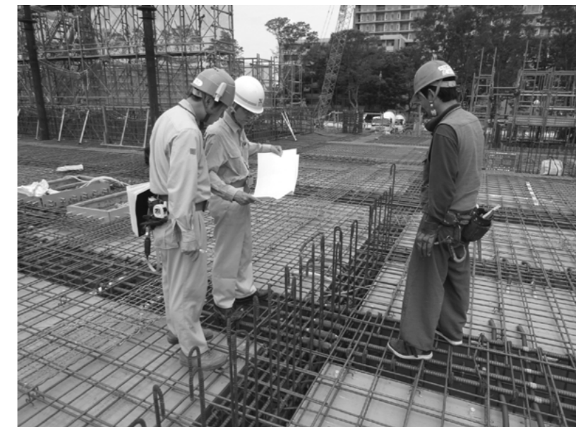
Figure 1. A bar arrangement inspection attended by the supervisor
