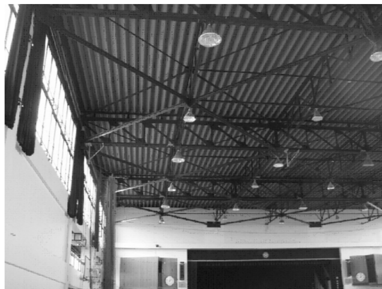
Figure 1. Seismic strengthening of gymnasium. Ceiling braces were replaced.
