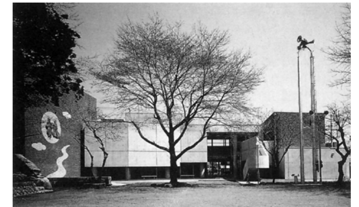
Figure 2. Tsukui Kushikawa Community Center (Kanagawa prefecture). A plaza integrated with the neighboring shrine ground provides a place to relax in everyday life, as well as functioning as a base for a community fire brigade, and is equipped with a wireless station for disaster prevention (photo: Akira Shimizu).
