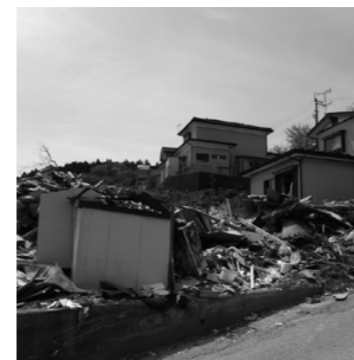
Figure 1. Housing sites on sloping land. Just a few meters of difference means a great difference in damage.
