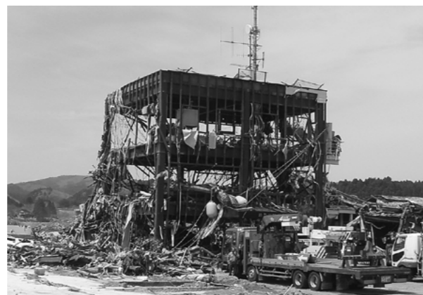
Figure 1. Whole of the disaster prevention building of Minamisanriku-cho, a 3-story steel frame building, was flooded by the tsunami and all of the ALC exterior walls and interior finishes were washed away. Only a few people who climbed a steel tower on the roof and were subjected to repeated tsunamis and snowing overnight survived.
