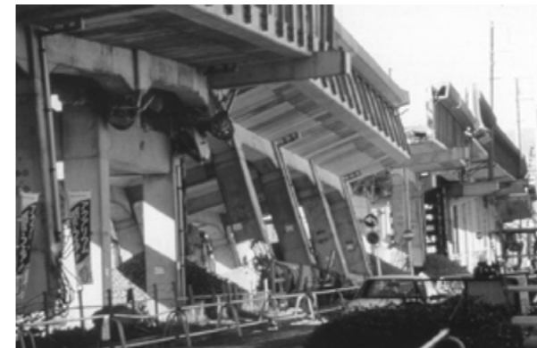
Figure 1. During the Great Hanshin-Awaji Earthquake, civil engineering structures and buildings suffered great damage, resulting in the public losing their trust in such constructions.
