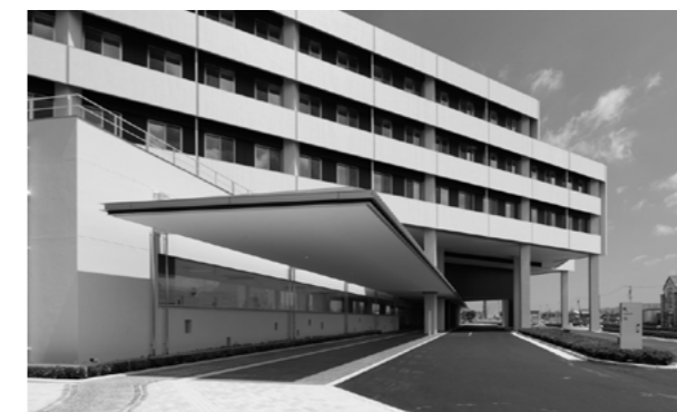
Figure 1. A large roof on pilotis designed with a triage function for use in an emergency (Ise Red Cross Hospital, Designed by Nihon Sekkei)
