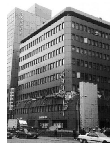
Figure 3. A steel encased reinforced concrete building, whose intermediate story with open web type columns collapsed
