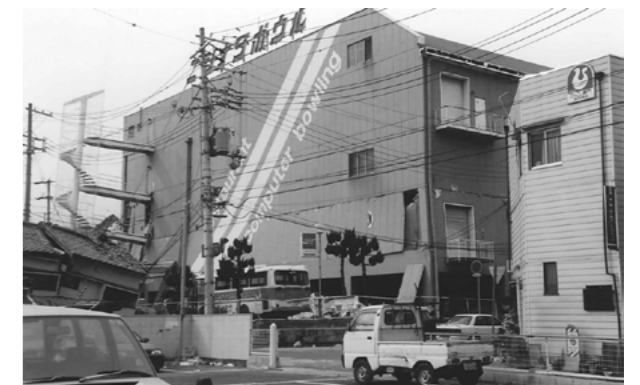
Figure 2. Collapse of an ALC panel (the Great Hanshin-Awaji Earthquake)
