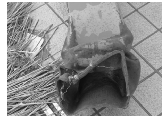
Figure 4. At the time of the Great East Japan Earthquake, many steel structures suffered damage; investigations into the validity of their construction methods need to be held.
