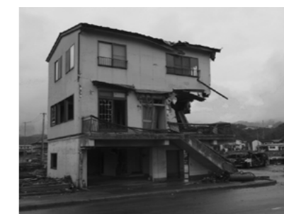
Figure 4. A mixed structure building with the ground first floor made with a reinforced concrete structure and the second and the third floors made with a wooden structure. Part of the second floor has been damaged by floating wreckage.
