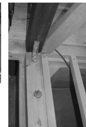
Figure 2. Addition of new foundation and sill, and strengthening a column base.
