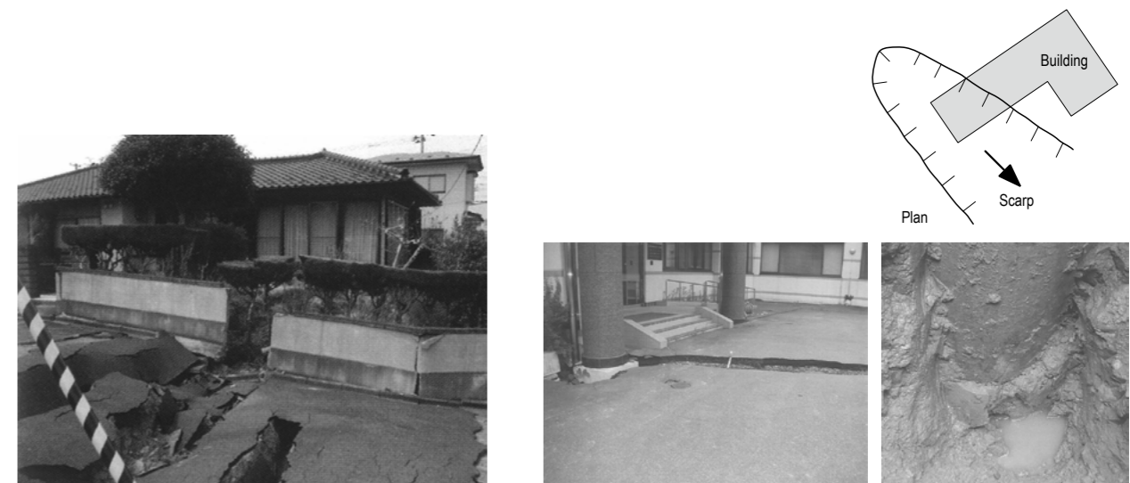
Figure 1. Damage to a valley filled building lot (Yamamoto-cho, Watari-gun, Miyagi prefecture, photo by Kazuya Mitsuji) 1)
