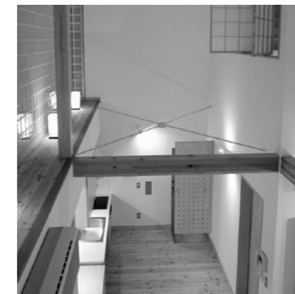
Figure 1. Ensuring horizontal rigidity with a catwalk and a horizontal brace
