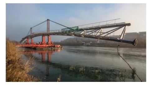
The installation operation meant a change in the structural system of the bridge from the assembled arrangement - a continuous beam structure with eight temporary supports - into a cantilever structure with temporary overhead cable support system. This system was necessary because of the low inertia of the section at the supports.
