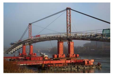
The entire structure to be moved was 160m long and 8m tall and the operation involved translating this structure horizontally by 30m on rails and onto two 60m-long barges which were coupled side by side, and on which temporary rails had been installed.
