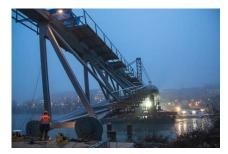
At the same time, the steel elements for the superstructure were fabricated in Aigle in Switzerland where steel manufacturer Z&M is based. The heavy-load truck transport was organised in three phases. The two ends of the main arch were assembled and welded on the site, after the single tube elements up to 16m long, diagonals and vertical diaphragm structures and upper box girder units were brought to the site by truck. The central third of the arch was brought to site in a single piece.
