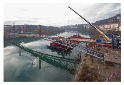
It was intended to minimise the time for which the river had to be closed to shipping traffic, and also offered the best solution for achieving geometrical accuracy during assembly on the site. Another benefit was that welding and coating operations were simplified with this procedure, and installation of equipment was made easier.
