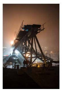
High performance jacks were used to lift the steel structure onto two Mammoet temporary supports, each consisting of two towers, and they moved the structure along a temporary rail system that had been built. The jacks were able to raise the structure about 2m higher than its final elevation; they had a capacity of about 500t per column, well above the 200t that was required.
